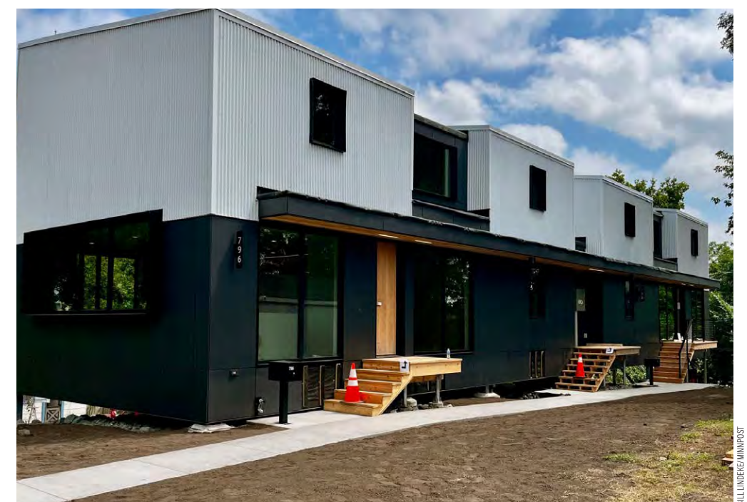
A new co-living duplex in St. Paul, where each unit will have six bedrooms and six bathrooms.
