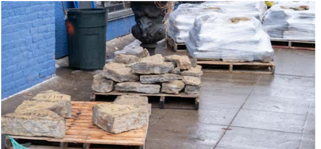
(above) Crews deconstruct the Justus Ramsey House, labeling the structure's stones that will eventually be reconstructed at a to-be-determined site. (right) Labeled stones from the Justus Ramsey House on pallets
