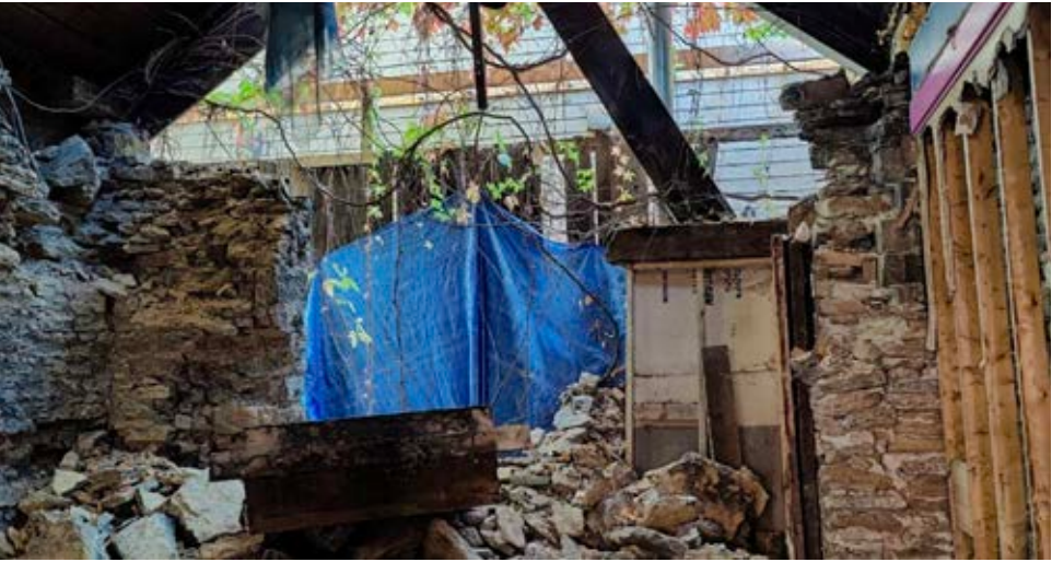
The collapsed eastern wall of the Justus Ramsey house is among the damage prompting the application for a demolition permit.
